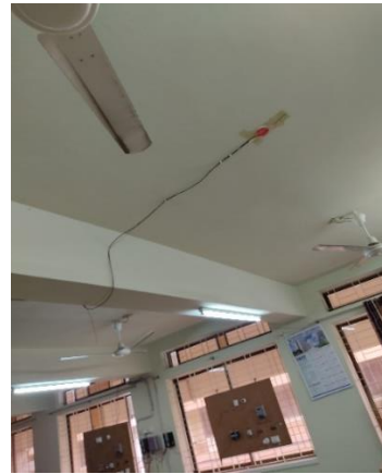
Fig.4 Heat flux sensors in the non air-conditioned room.
