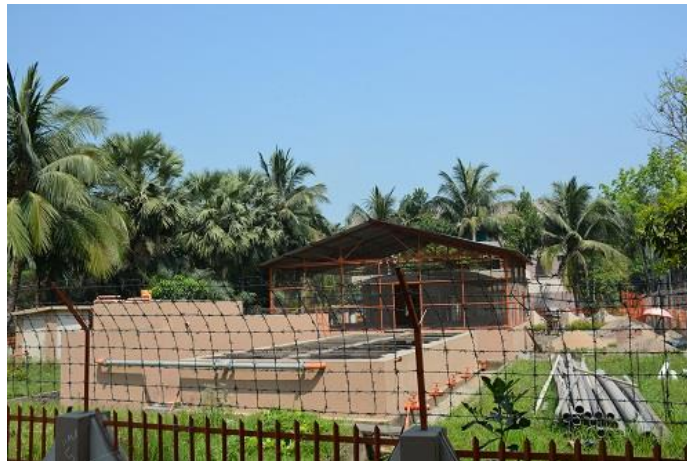
Figure 5: Water Treatment Plant KUET
